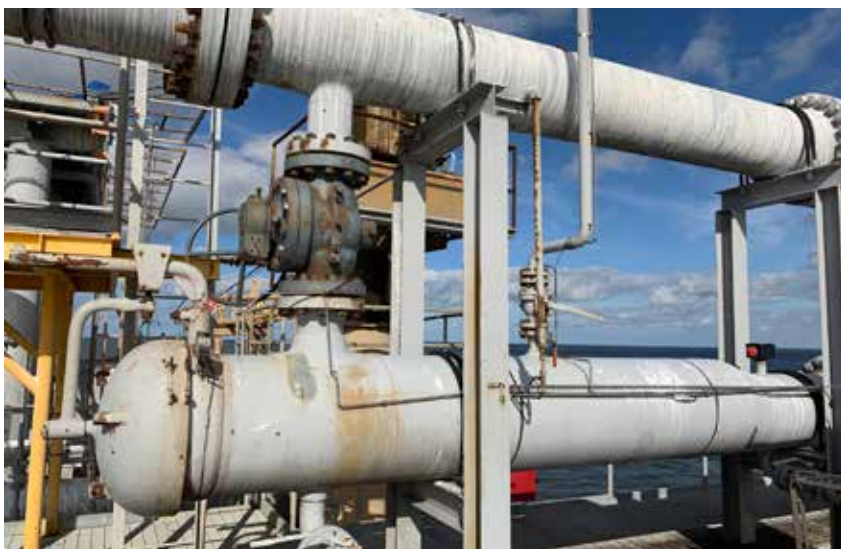
Platform jointly owned by Kinetica and Contango, set up to receive a pig that was launched from a production platform to remove condensates. Photo credit: Barney Paternostro
